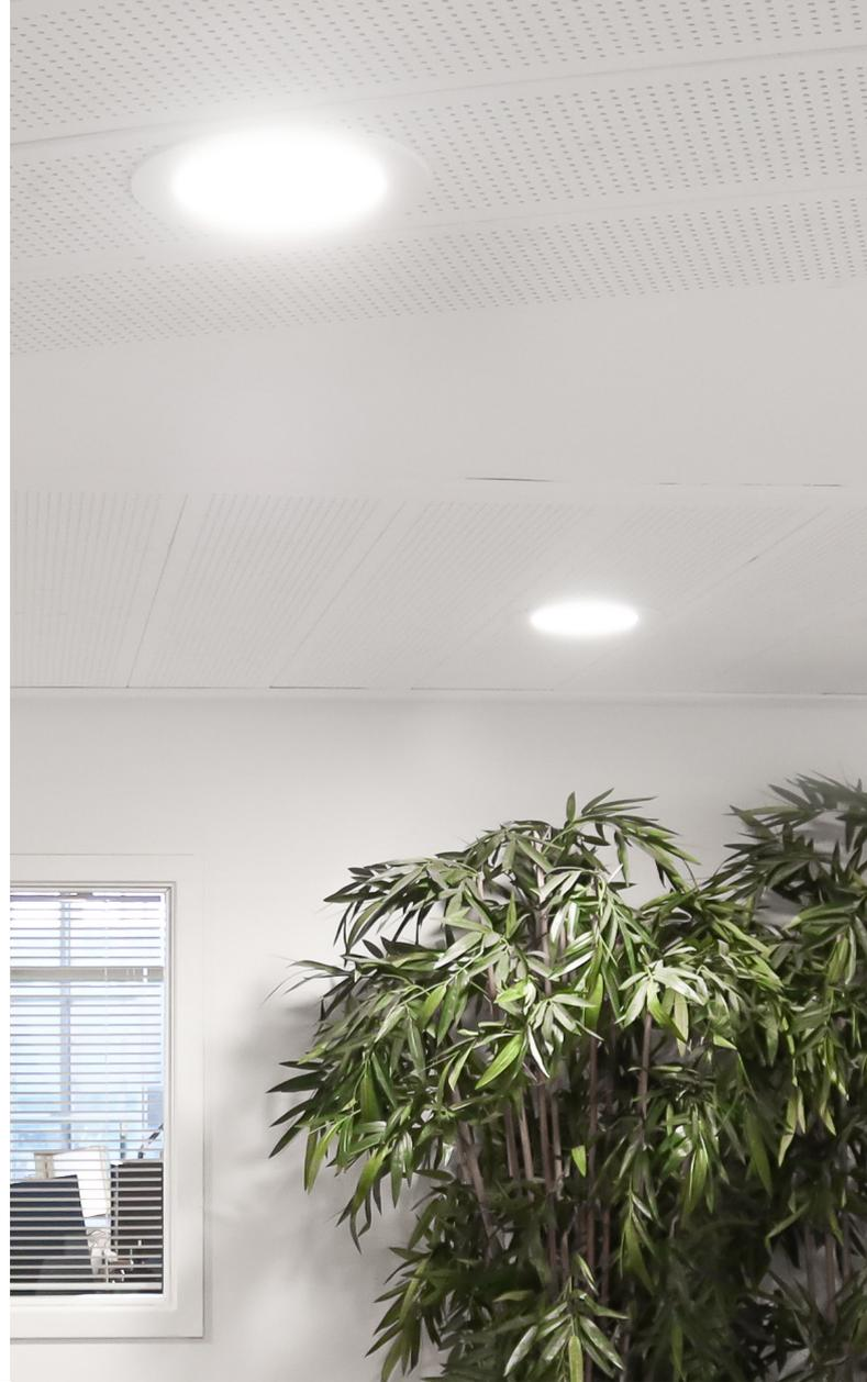
**PerfectFit has made it much easier to renovate. With PerfectFit, the downlight is printed based on specific measurements, so that there is no need for extra trims, to adapt the downlight to the cut-out.**
